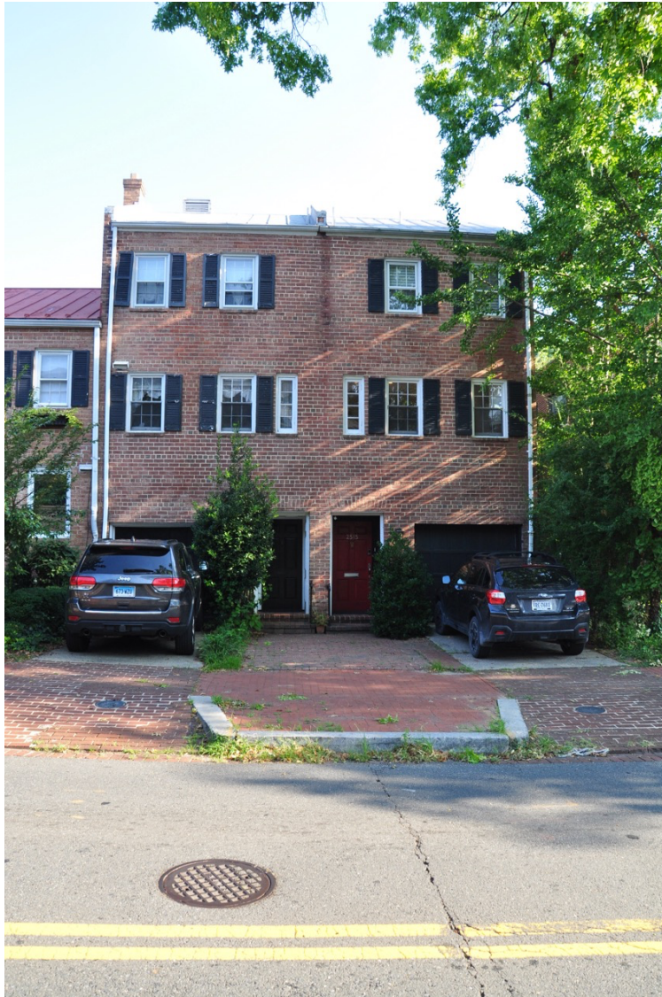
Front Elevation (2517 at left) Looking North
