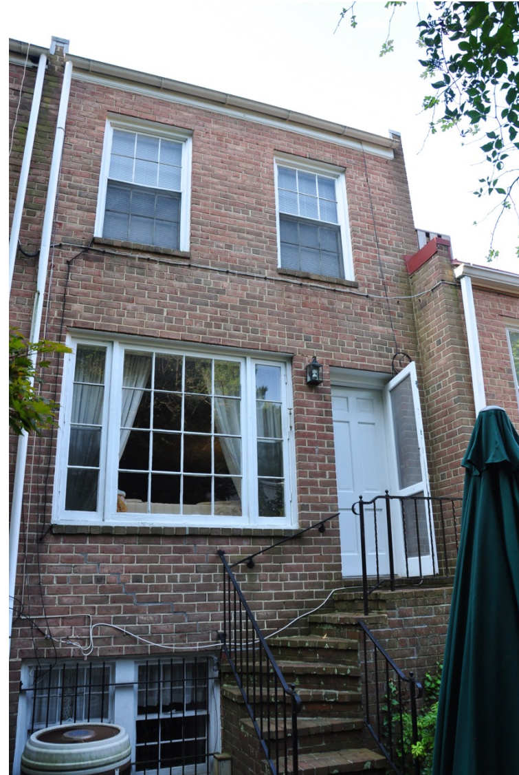
Rear Elevation Looking South
